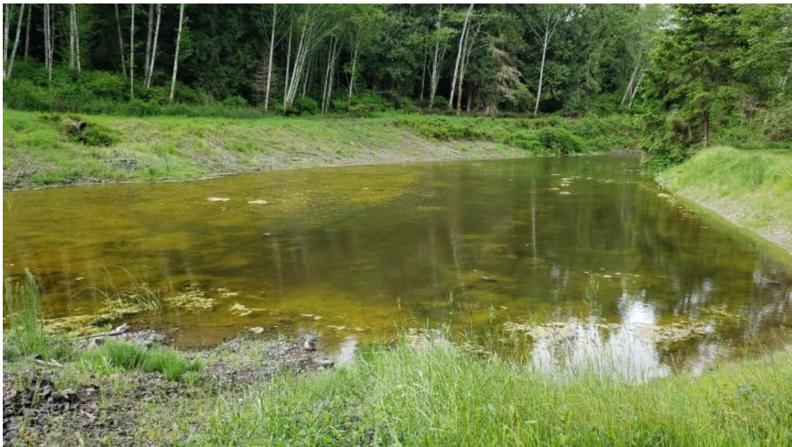
General Site - Stormwater, Pond, Renovate
