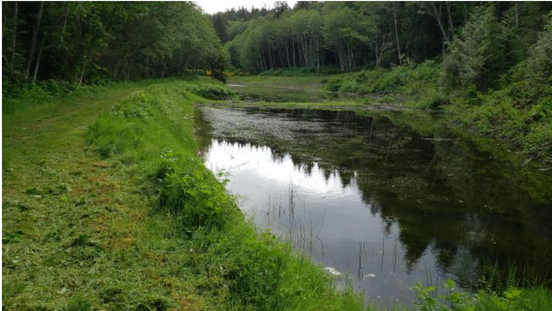
General Site - Stormwater, Pond, Maintain
